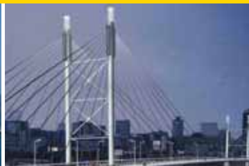
Ponte Nelson Mandela
